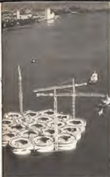
STORAGE TANKS OFF NORWAY More troubles than benefits.
