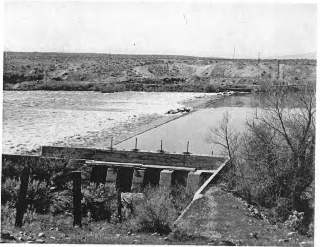
Diversion dam on Yakima River. Gates at near end serve the Richland Irrigation District; those at far end serve the Columbia Irrigation District.
